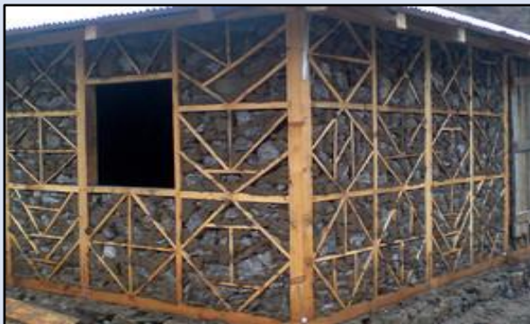
Reinforcement of Traditional Housing Structures Using Timber and Masonry Techniques
