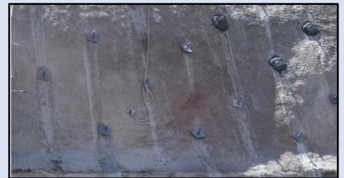
Ground Anchor Wall with Riprap and Shotcrete Slope Stabilization
