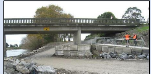
Scour Protection Using Concrete Block Armoring Around Bridge Piers
