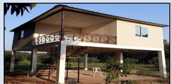
Elevated Housing on Stilts for Flood-Resilient Construction in Low-Lying Areas
