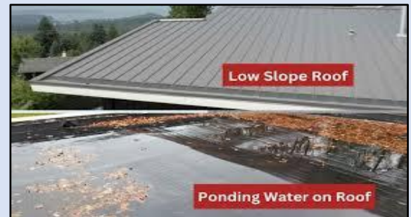
Sloped and Pitched Roofing Systems for Improved Rainwater Drainage
