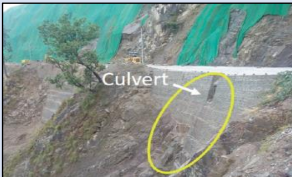
Culverts and Aqueducts for Hydraulic Capacity Enhancement
