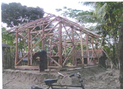
Figure 4: Reinforced frame of a house in Noakhali and the completed house
