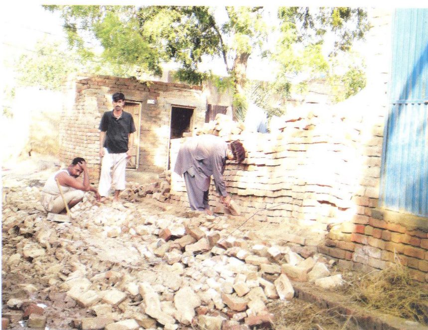
Boundary wall of a house collapsed due to heavy rains in Muzaffargrh, is being repaired.
