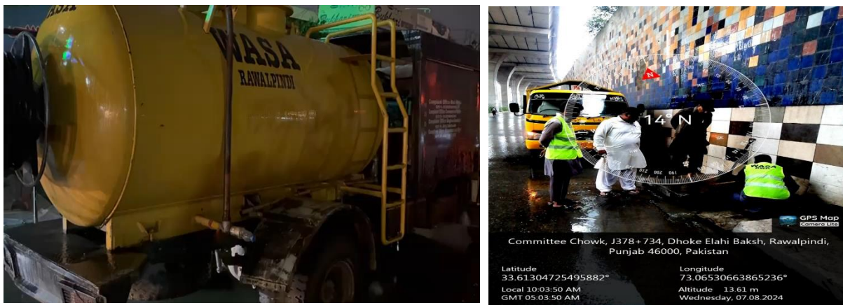
Figure 3.10. Dewatering at Liaquat Bagh and Committee Chowk, Rawalpindi
