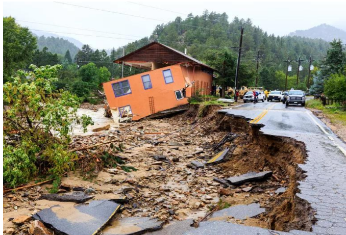
Figure 6.2. Structural damages due to urban flooding
