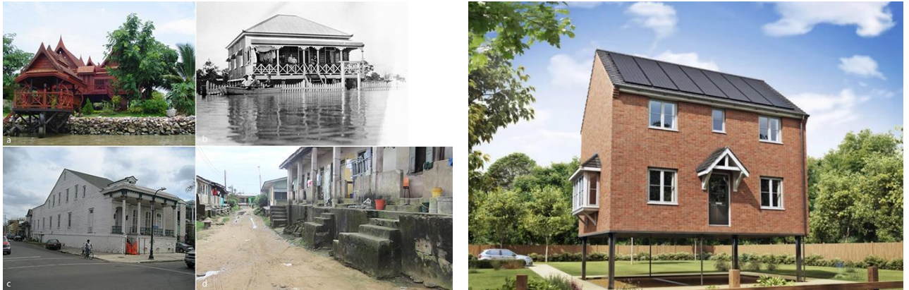
Figure 8.13. Flood resistant buildings
