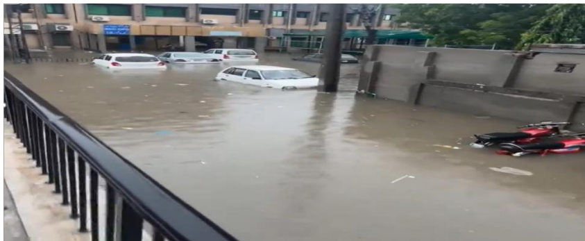
Figure 3.8. Urban flooding in Services hospital Lahore -- Aug 2024
