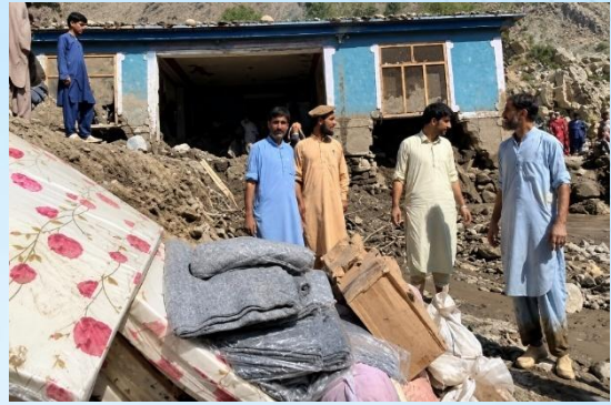
Figure 17: Residential damage intensified by encroachment on natural waterways
