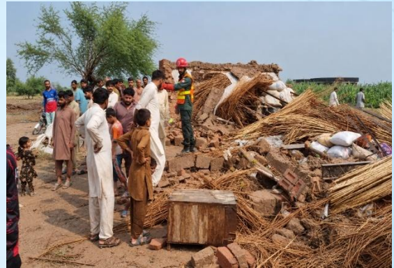
Figure 14: Flood-damaged house constructed with substandard masonry materials, showing severe wall deterioration and fully collapse.
