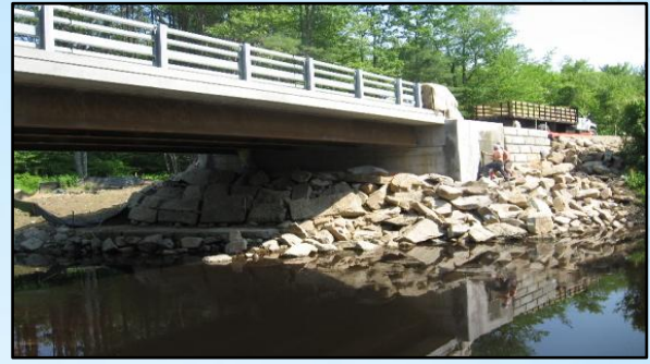
Figure 36: Riprap protection installed to resist erosion at an embankment or channel bank.
