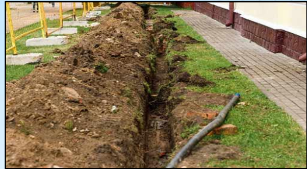
Figure 40: Maintenance of a local surface drain to prevent water accumulation near structures.
