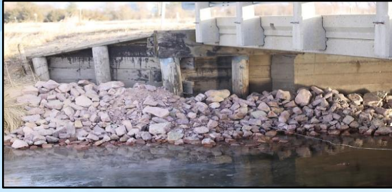
Figure 51: Riprap protection installed at a bank or structure foundation exposed to sustained flood flow.
