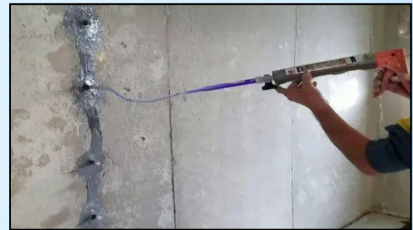
Figure 42: Epoxy injection repair of a structural crack in masonry.
