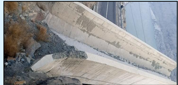
Figure 54: Aqueduct structure illustrating conveyance design across a flow path.
