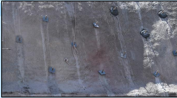
Figure 27: Ground anchor wall installation providing lateral slope stabilization.
