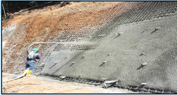
Figure 43: Shotcreting application on an exposed slope or structural surface for erosion protection.
