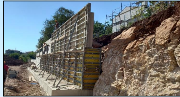
Figure 28: Retaining wall construction protecting an embankment or road edge from erosion.
