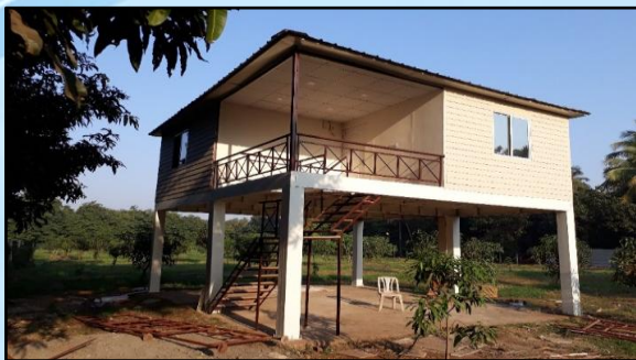
Figure 63: Elevated housing construction reducing exposure to flash-flood inundation.
