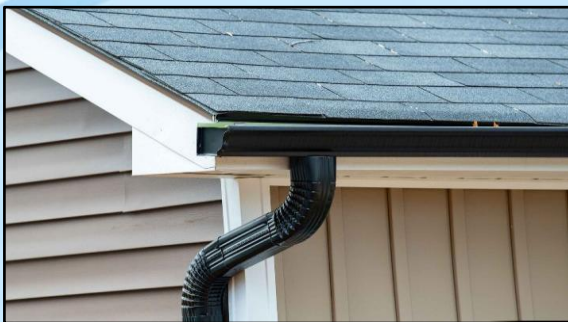
Figure 55: Site grading and drainage provision directing runoff away from a residential structure.
