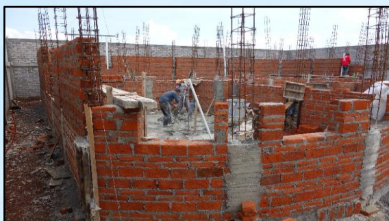
Figure 57: Reinforcement of a housing structure to improve load-carrying capacity.
