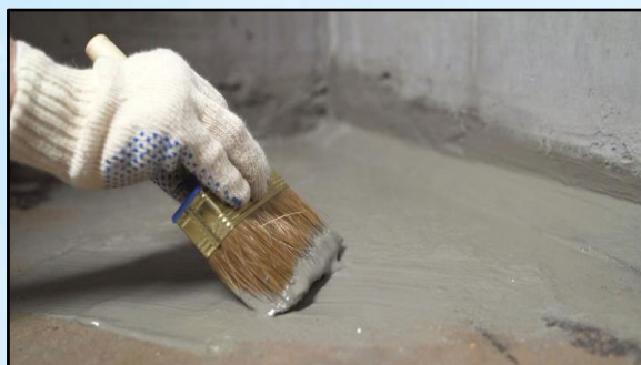
Figure 65: Cement-based waterproofing application on a residential structure.
