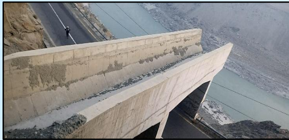
Figure 53: Aqueduct structure maintaining hydraulic conveyance across an intersecting alignment.
