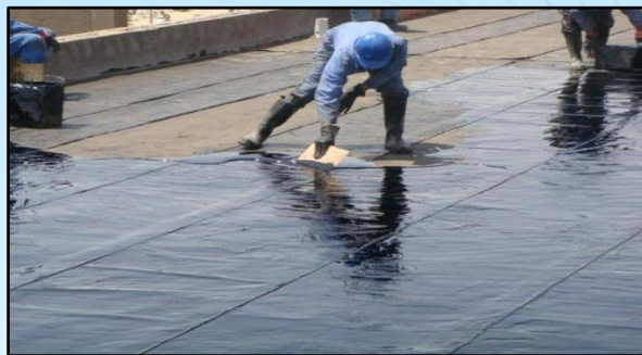
Figure 32: Bituminous coating application providing a waterproof membrane on exposed surfaces.
