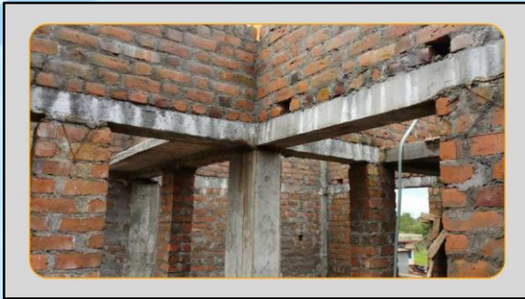
Figure 39: Band beam and column reinforcement integrated into residential masonry construction.
