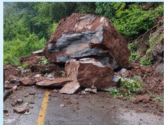
Figure 24: Soil erosion and landslide debris causing road embankment failure and disrupting connectivity during monsoon rainfall.
