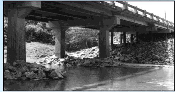
Figure 44: Riprap protection at a vulnerable embankment or channel bank.
