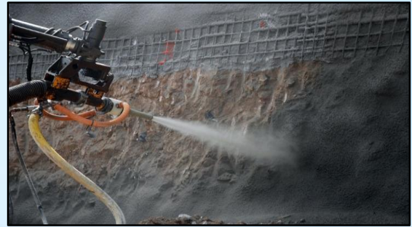
Figure 38: Shotcreting application stabilizing an exposed slope or structural surface.
