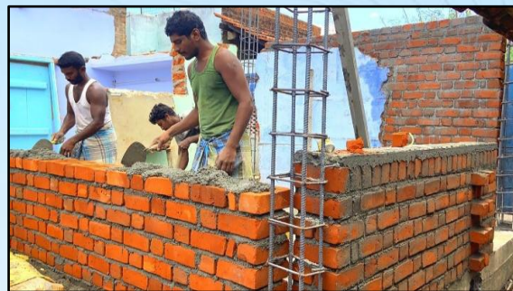
Figure 56: Reinforcement measures applied to improve residential structural resilience.
