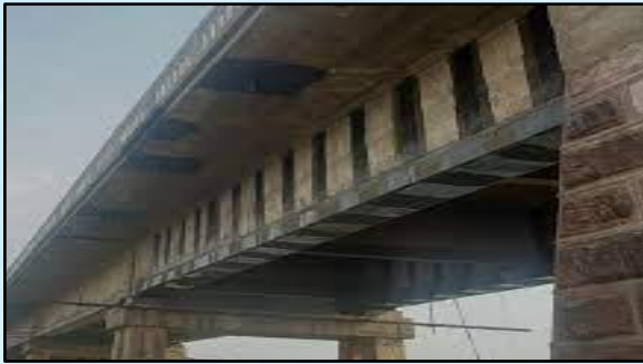
Figure 37: Structural bracing providing lateral stability to a vulnerable element.
