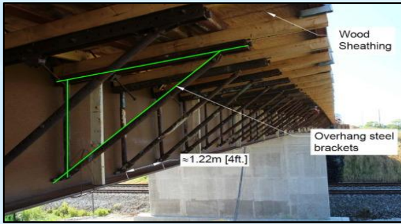
Figure 45: Structural bracing applied to a vulnerable communication infrastructure element.
