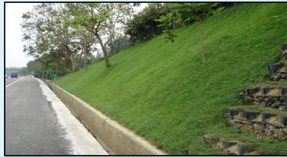
Figure 46: Slope vegetation used to stabilize exposed terrain and reduce surface erosion.
