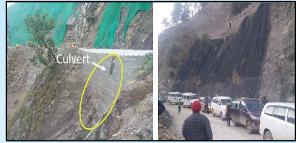
Figure 52: Culvert structure providing cross-drainage conveyance beneath a transport corridor.
