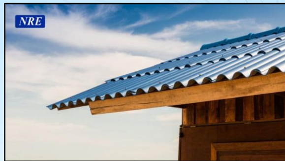
Figure 64: CGI sheet roofing providing rapid rainwater shedding.
