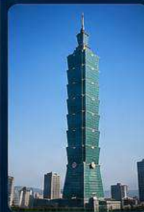
TAIPEI 101 Taipei, Taiwan World's largest TMD (660 ton)
