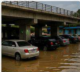
Mall Parking Flooding
