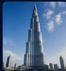
BURJ KHALIFA Dubai, UAE Central core shear walls provide exceptional lateral stability.
