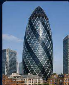
30 ST MARY AXE London, UK Diagrid structure for stability & efficiency.
