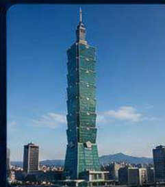
TAIPEI 101 Taipei, Taiwan Reinforced concrete core walls resist typhoon and seismic forces.
