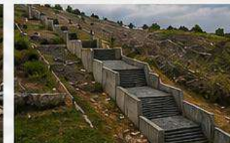
Slope Protection & Retaining Structures
