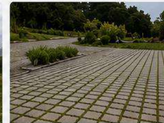
Permeable Pavements & Proper Drainage
