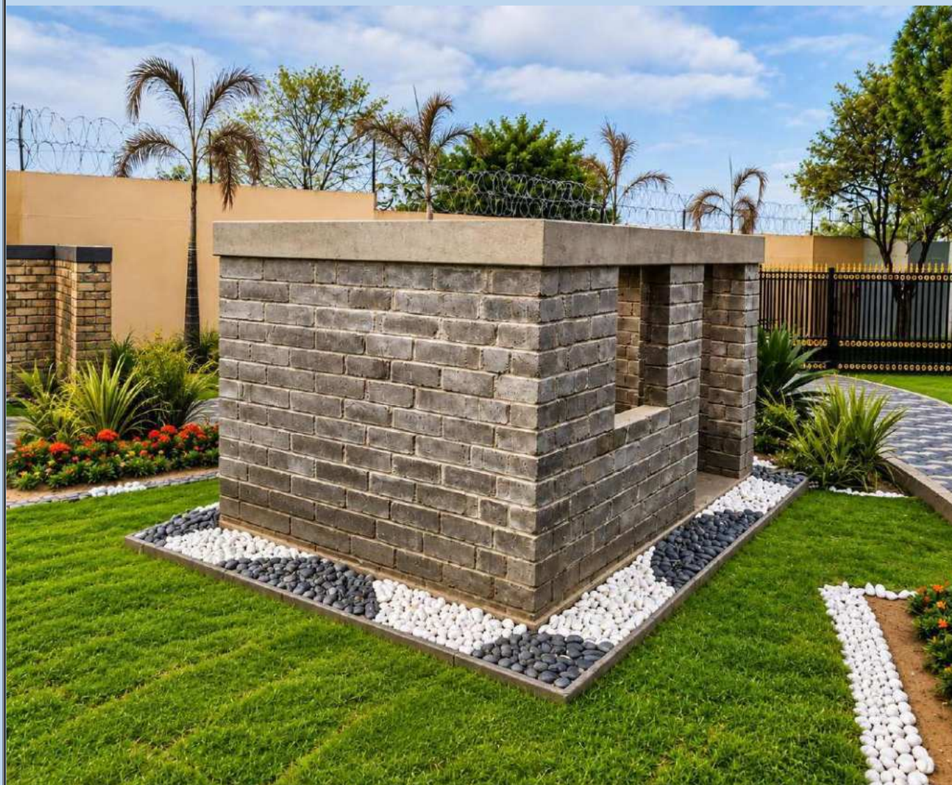
HP3 — Fly Ash Masonry Structure displayed at NDMA Headquarters, Islamabad
