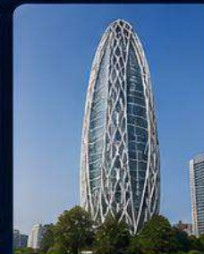
COCOON TOWER Tokyo, Japan Combines diagrid for strength & aesthetics.
