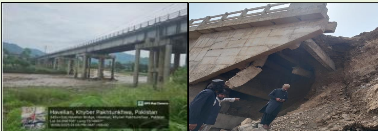
Figure 55: Structural Failures Due to Inadequate River Training and Scouring at Bridge Piers and Abutments
