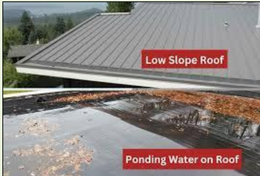
Figure 64: Sloped and Pitched Roofing Systems for Improved Rainwater Drainage
