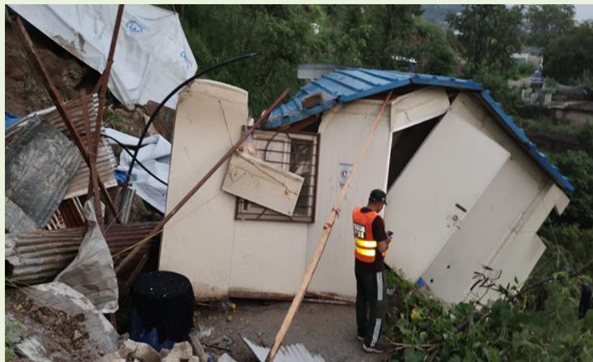
Figure 42: Structural Collapse of a Residential Unit in Muzaffarabad Due to Poor Site Selection
