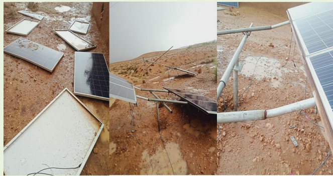
Figure 22: Solar Infrastructure Damage due to Heavy Rainfall
