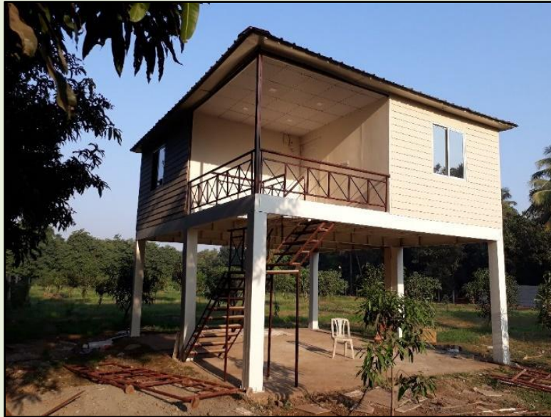
Figure 66: Elevated Housing on Stilts for Flood-Resilient Construction in Low-Lying Areas
