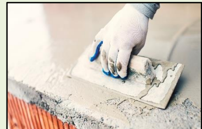
Figure 60: Application of Cementitious Waterproofing for Enhanced Structural Durability
