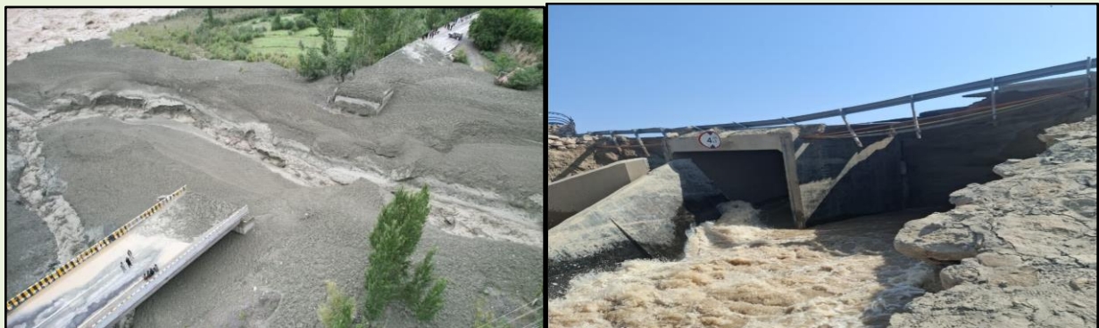
Figure 56: Structural Impacts of Sedimentation and Debris Load on Bridge and Culvert Systems
