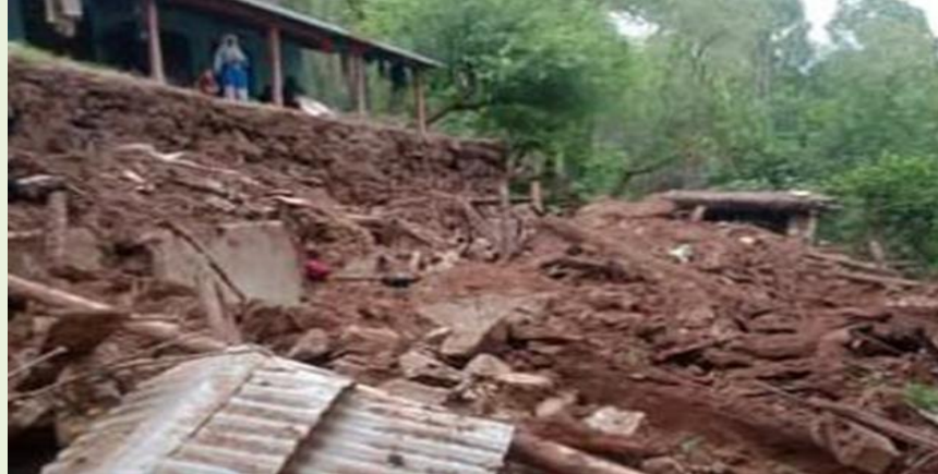
Figure 41: Structural Collapse of Residential Buildings in Sudhnoti Due to Weak Design and Materials
