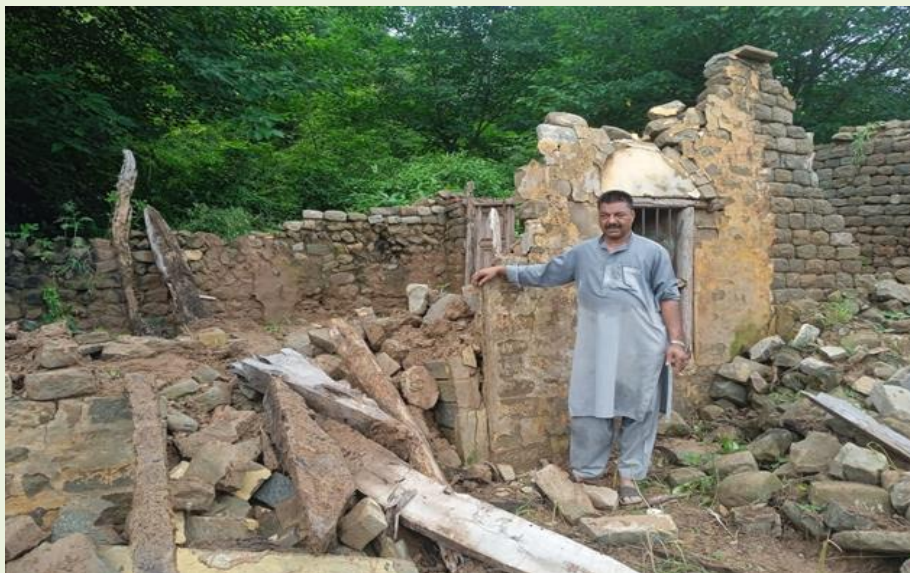
Figure 46: Structural Failure of an Aged Residential Unit in Mirpur Due to Lack of Maintenance
