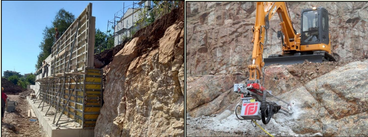
Figure 67: Slope Stabilization Techniques – Construction of a Retaining Wall (left) and Application of Soil Nailing (right) for Slope Reinforcement.
