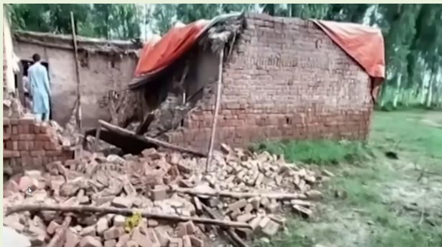
Figure 13: Structural Collapse of Residential Houses in Sargodha Due to Poor Construction Practices
