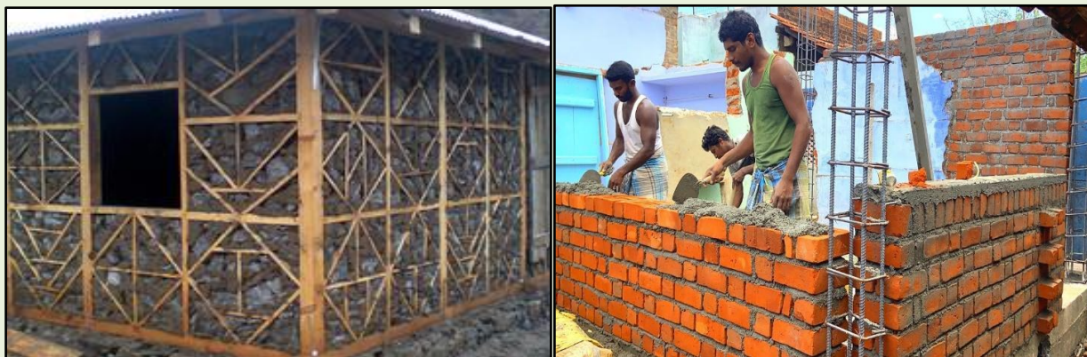
Figure 65: Reinforcement of Traditional Housing Structures Using Timber and Masonry Techniques
