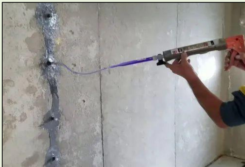
Figure 63: Epoxy Injection for Structural Crack Rehabilitation
