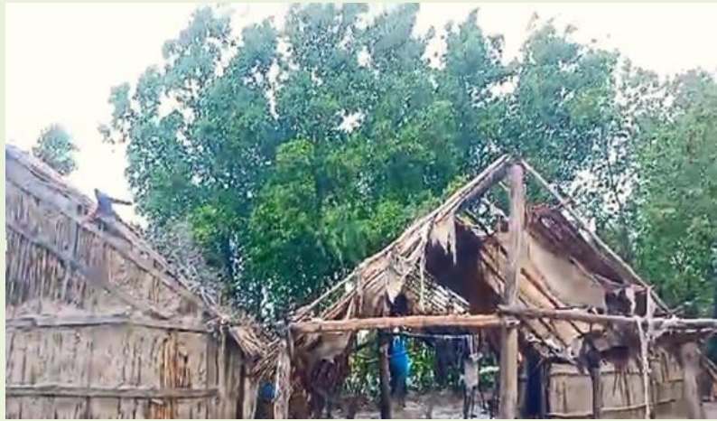
Figure 31: Mud and Thatch House Damage due to Flash Flooding Triggered by Intense Monsoon Rainfall
