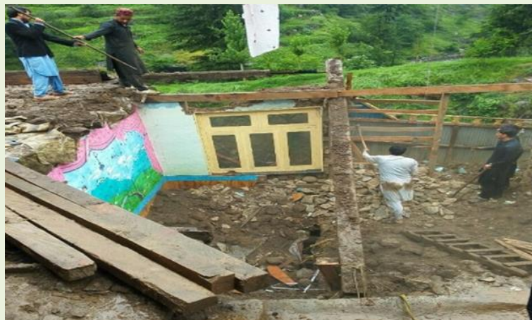
Figure 6: Roof Collapse Due to Rainwater Accumulation
