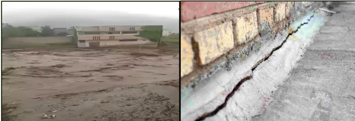
Figure 52: Foundation Failure and Structural Cracking Caused by Poor Drainage and Soil Instability
