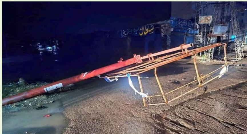
Figure 10: Failure of Unbraced Electrical Pole Infrastructure
