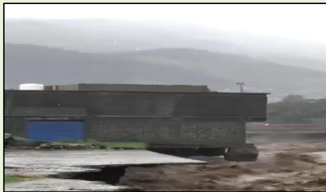
Figure 47: Structural Instability Caused by Foundation Soil Erosion
